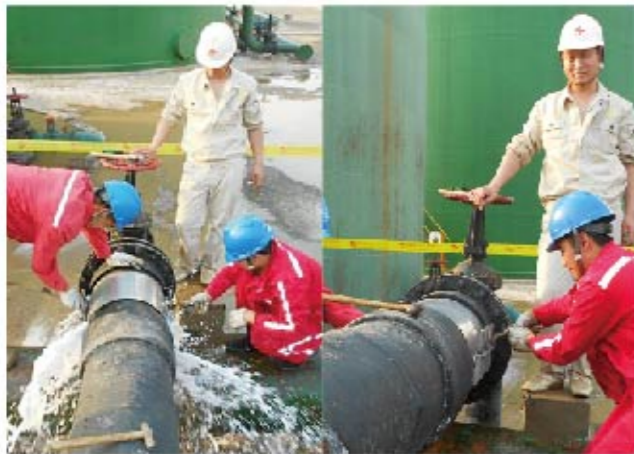
Within 3 minutes, under pressure leakage repairing has done successfully on the DN450 water supply pipeline in Puyang Oilfield.
