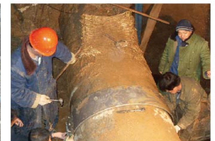
RCD Double-Section Repair Clamps apply to the DN1200 cement pipe.
