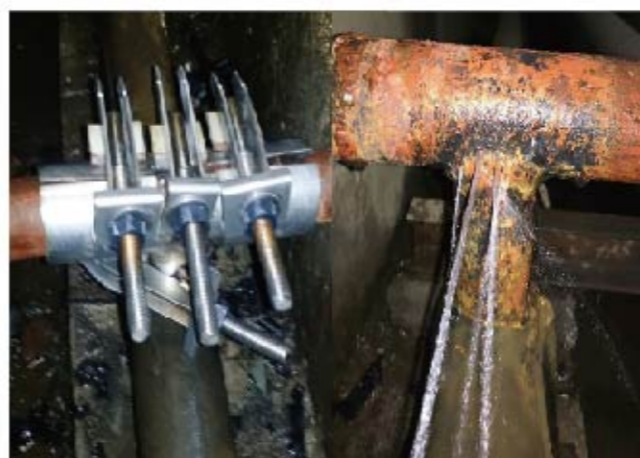
Zhuhong Tee Clamp functions very well on the tee part of DN40 pipelines in the High Railway Station.
