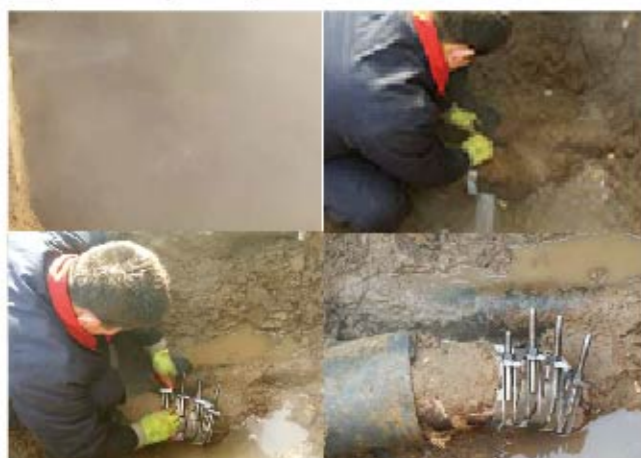
Within 10 minutes, Zhuhong Elbow Repair Clamps have been used to repair the 90° degree elbow of DN150 steel pipe.
